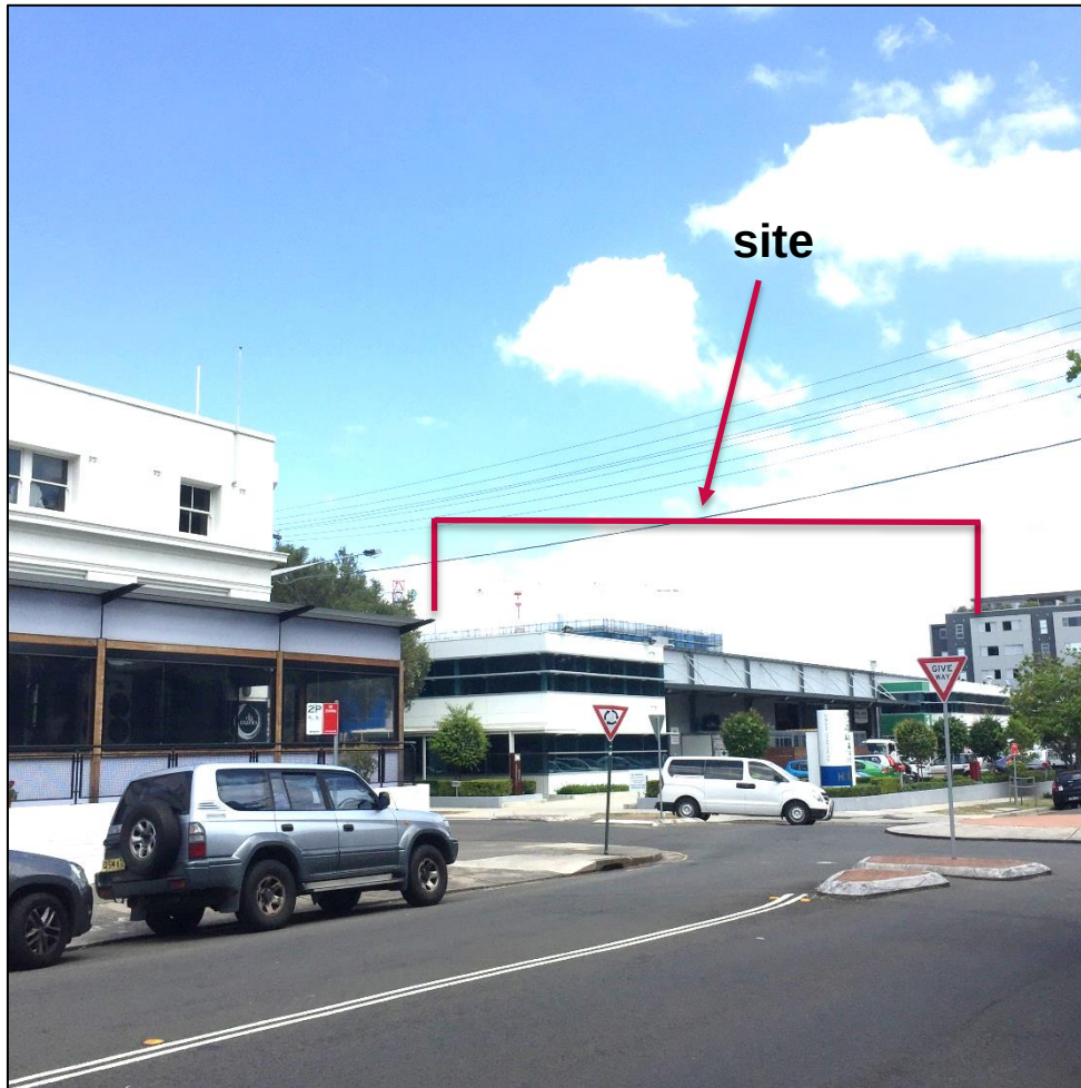
Figure 4 The site as viewed looking south west from Morley Avenue. 36 Morley Avenue in foreground.
