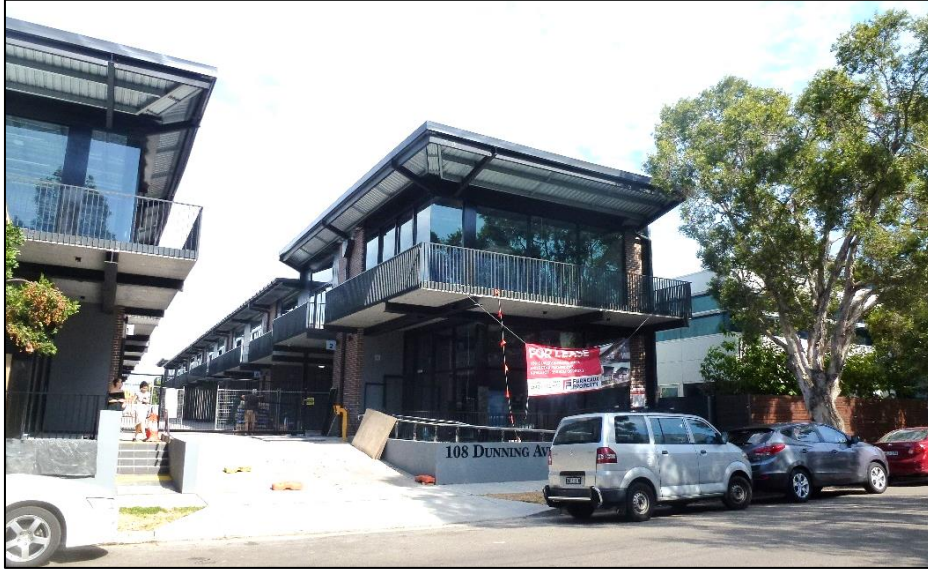
Figure 8 Recent development on 108 Dunning Avenue, Rosebery
