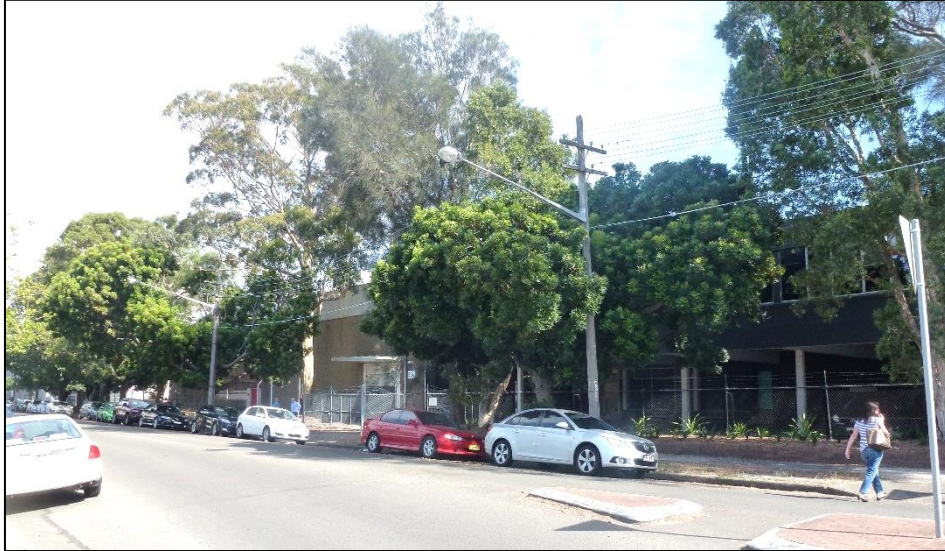
Figure 6 Existing two-storey light industrial warehouse at 33-35 Morley Avenue
